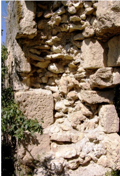
Fig. 6: Internal structure of the southwestern wall of the fortress Skivarin.
