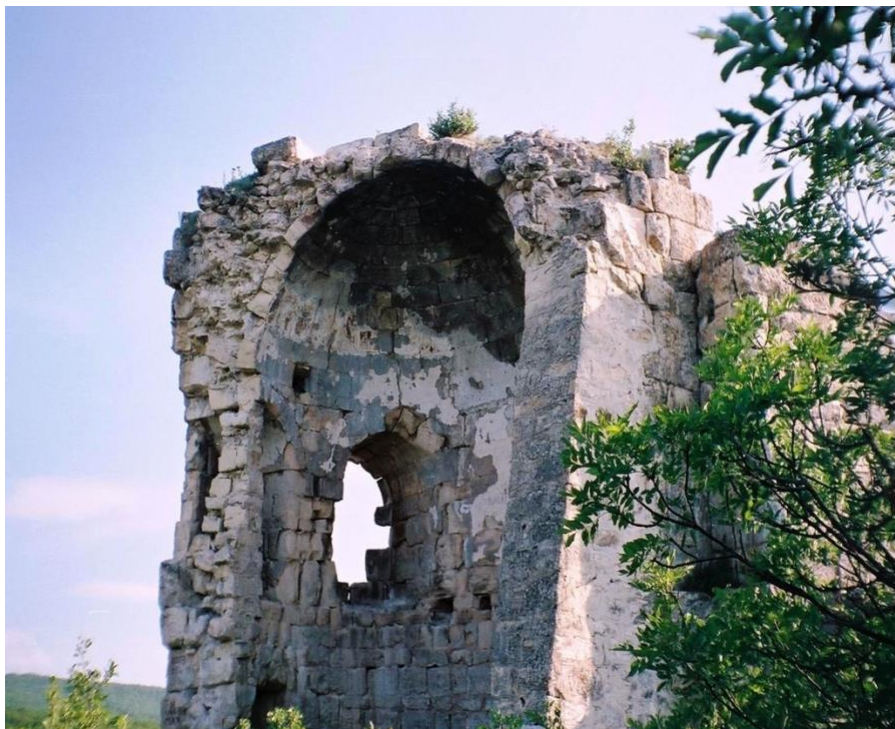
Fig. 9: Tower of the fortress of Skivarin, view from the inside.
