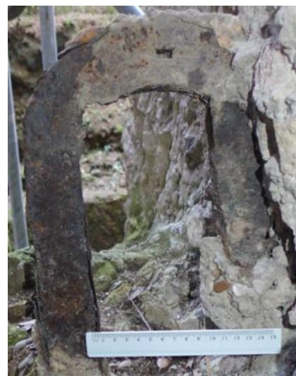
Figure 4b. U-shaped bracket still embedded in masonry seen from the East (Photo A.).
